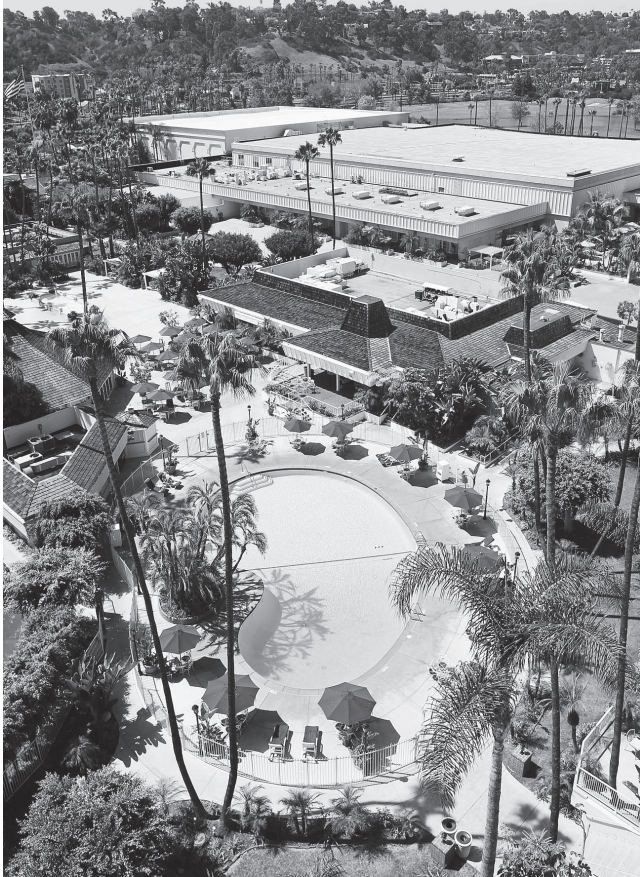
A major renovation is planned at the Town and Country Resort & Convention Center. K.C. ALFRED • U-T
